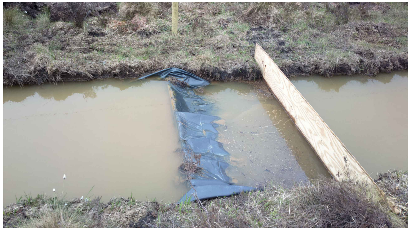
Baffle/Weir Detail
