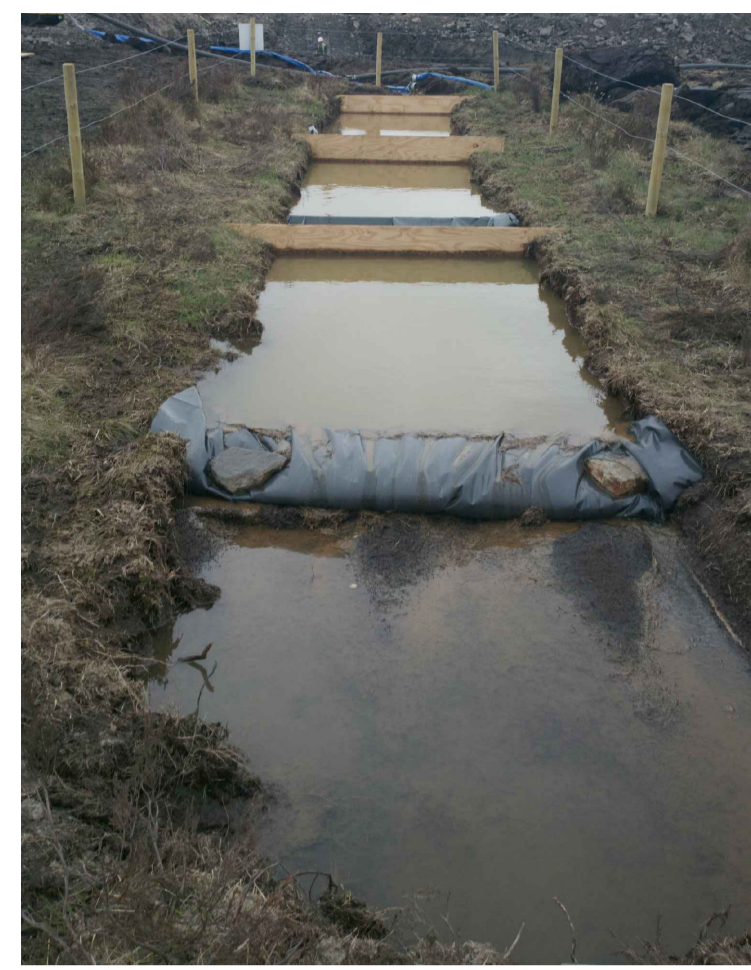
Completed Settling Pond System
